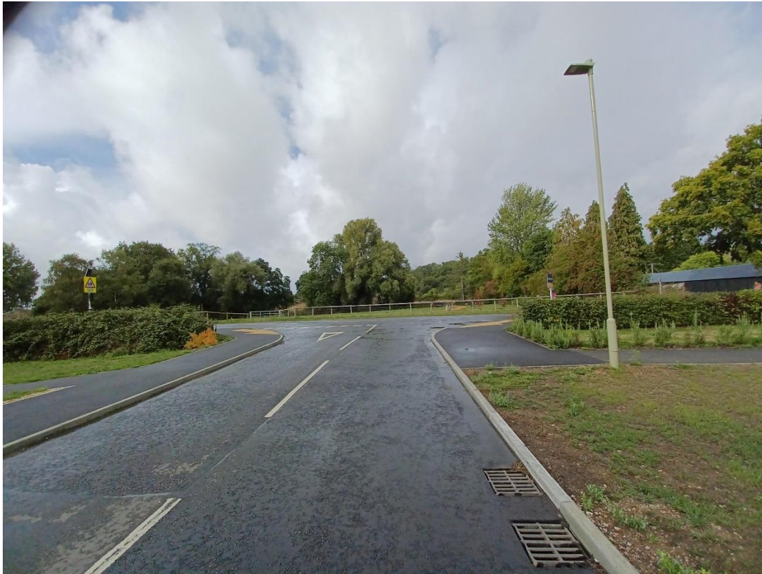
Looking towards Whitsbury Road and point of new roundabout and site access from Augustus Park
