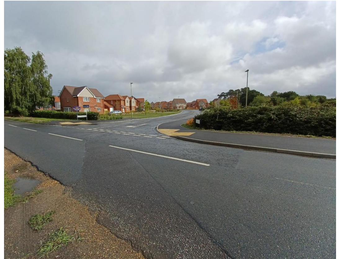
Site of new roundabout and current entrance to Augustus Park
